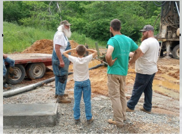
Well drilling in progress
