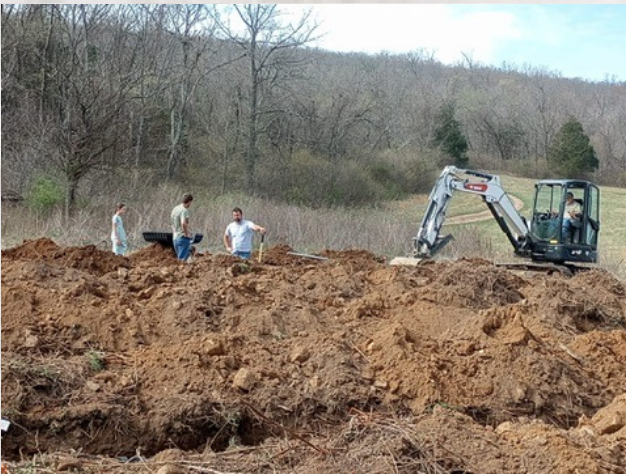
Installing field lines for the septic system
