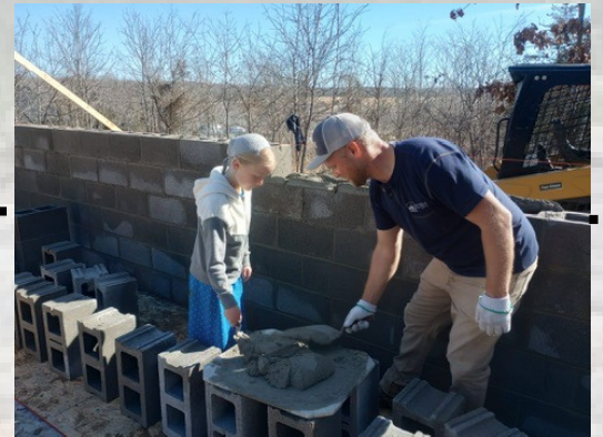
Volunteers laying block for the shower house
